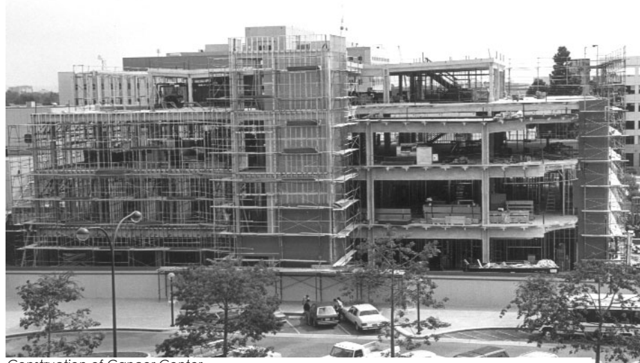
Construction of Cancer Center
