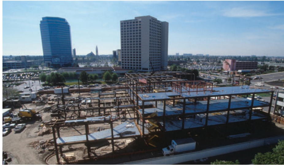
Construction of UCI Neuropsychiatric Center
