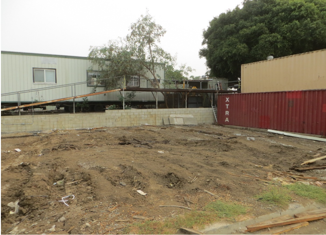
Photograph 5: A portion of the permanent footprint contains structures and facilities, increasing the amount of disturbance present.
