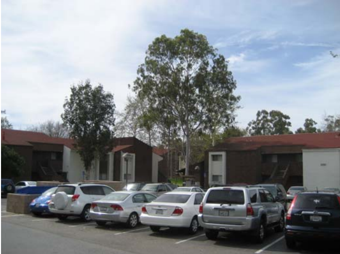
4. Southwest into project site from Adobe Circle Road South
