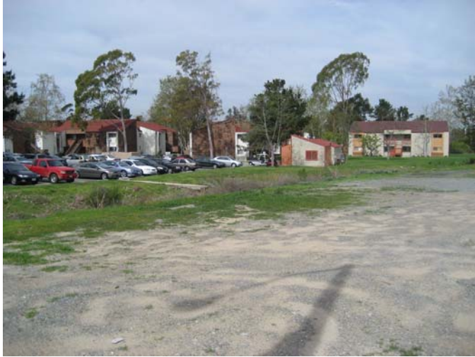
7. Northwest towards project site from California Avenue
