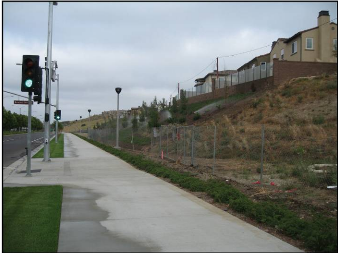
9 Toward adjacent faculty and staff housing, under construction
