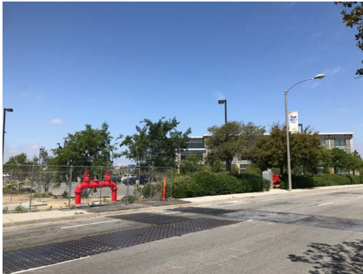
View 1: Southern boundary of the project site looking northeast toward the project site and Gavin Herbert Eye Institute.
