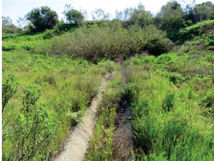
View looking southwest at Basin 1 and V-ditch B1B, (2/28/2017).
