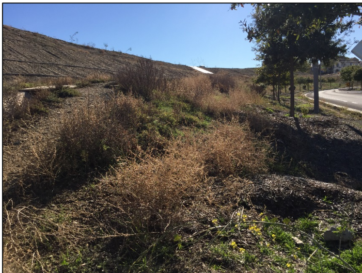
View 6: Northeast corner of project site looking southwest toward project site along California Avenue.
